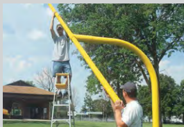
Tip Crossbar to Level and Clamp
